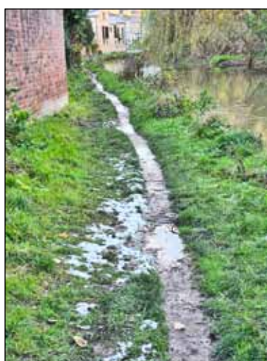
Left: before repairs
