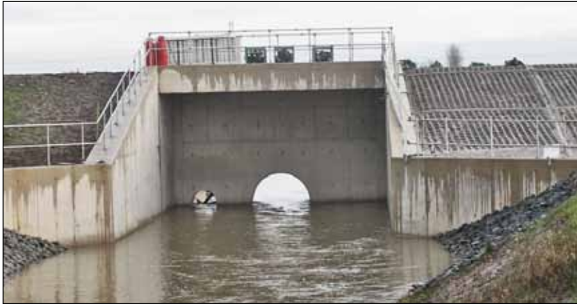
The newly constructed flood barrier
