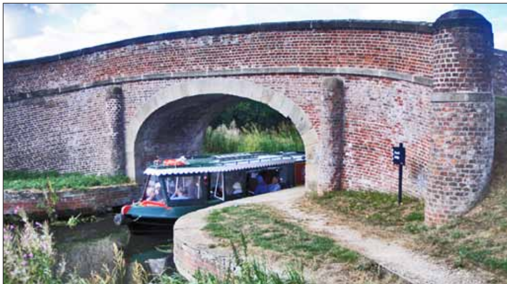
Church Bridge, Melbourne. Architecturally one of the best bridges on the canal system.
