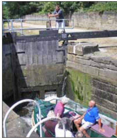
Rather than using a windlass a wooden spike is used to open many locks on the C&H Navigation
