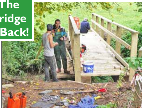
Conservation Volunteers at work on the footbridge
