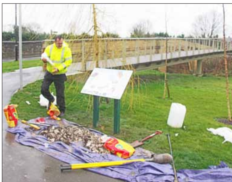
Installing the board
