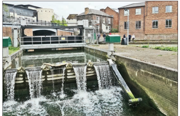
The weir at Castle Mills shows the eel pass on the right
