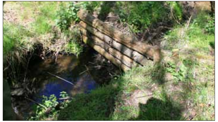
A 'leaky dam', part of NFM at Pickering
