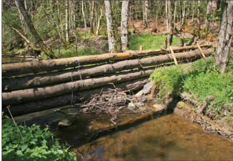
One of Pickering's 'leaking' dams
