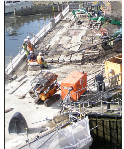
Works during summer 2011
